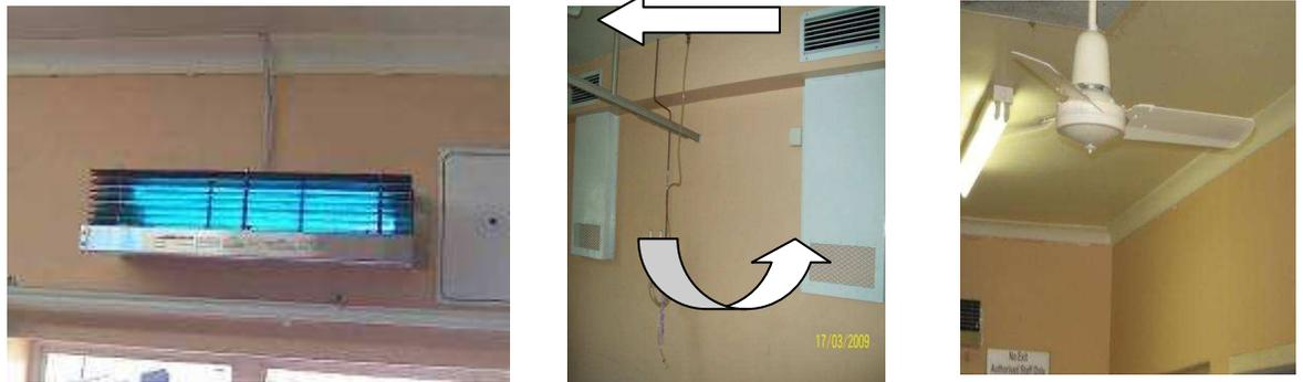
**Figure 2:** a) UVGI wall fixture, b) room ventilation arrangement, and c) ceiling paddle fan model in use during experiments. *Note that the photo 2a was taken wearing UV protective goggles as even brief direct exposure at close-range to upper room UVGI lamps can cause corneal inflammation.*
